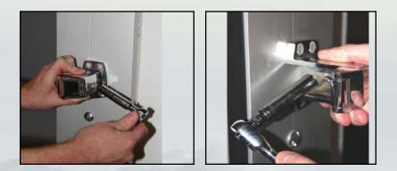
The strike roller is fully retracted and must be adjusted out by the installer.
