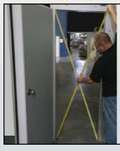
Measure the opening diagonally to make sure door assembly is set square in opening.
