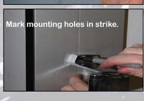
25. Close door and set roller assembly. Use a 9/16" socket and remove inside and outside bolts. Slide roller assembly section of strike out. Insert bolt in hole furthest away from strike base. Set strike so door is snug and tighten outside bolt. On the inside of the roller assembly insert bolt in outer hole and tighten bolt.
